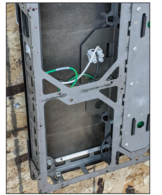
Figure 8: Install Power Entrance
