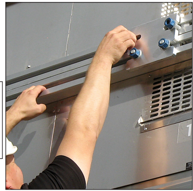
Figure 13: Attaching Splice Plate
