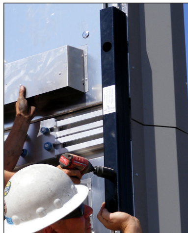
Figure 15: Aligning and Installing the Vertical Splice Tubes
