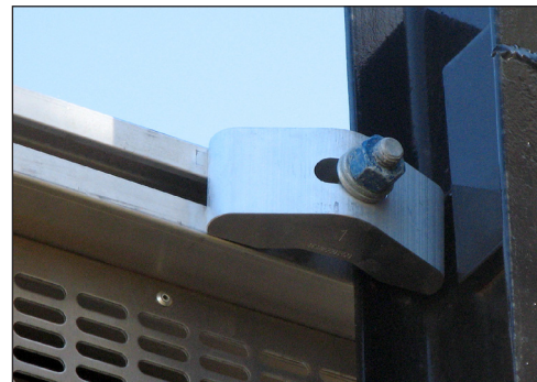
Figure 5: Rocker Clamp Engaging Upright
