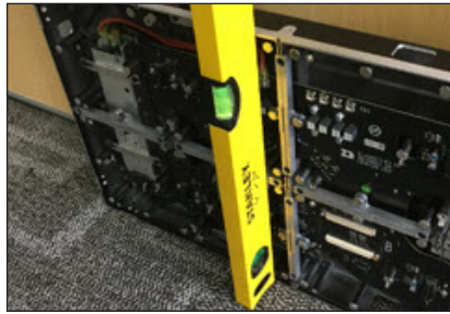
Figure 22: Ensure Panel is Level and Vertically Plumb
