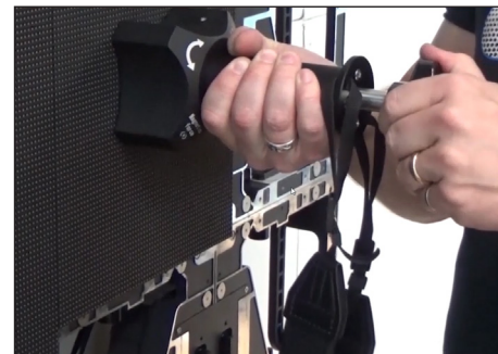
Figure 23: Remove Module
