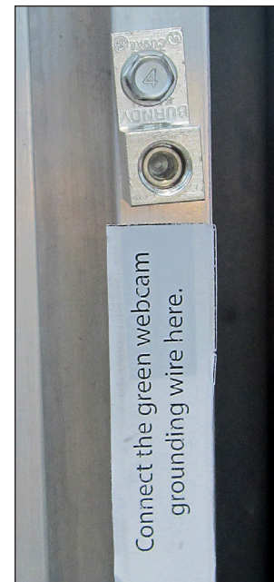
Figure 25: Webcam Grounding Lug
