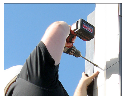
Figure 17: Attaching Vertical Splice Cover
